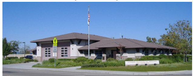
Fire Station 8 5750 Scenic Avenue (Livermore)
