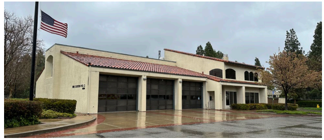
Fire Station 2 6300 Stoneridge Mall Road (Pleasanton)
