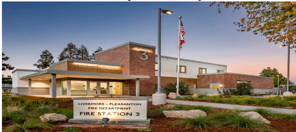
Fire Station 3 3200 Santa Rita Road (Pleasanton)
