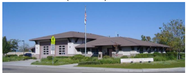
Fire Station 8 5750 Scenic Avenue (Livermore)
