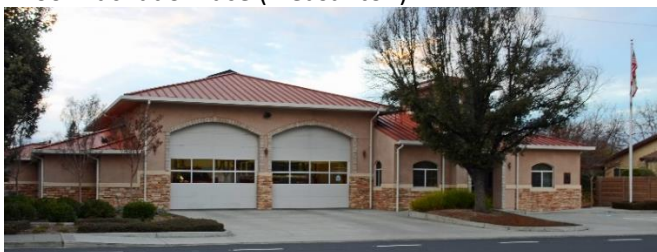
Fire Station 7 951 Rincon (Livermore)
